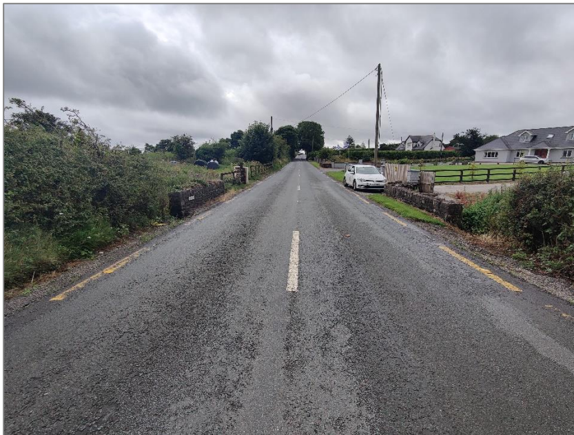
Figure 5 - Bridge B3/C3 towards Dungarvan Substation [WD-R672-003.00]
